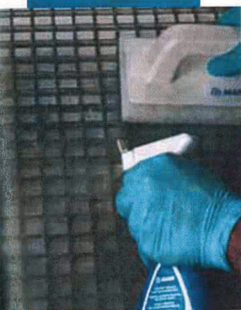
Spraying Kerapoxy Cleaner on the surface requiring cleaning
