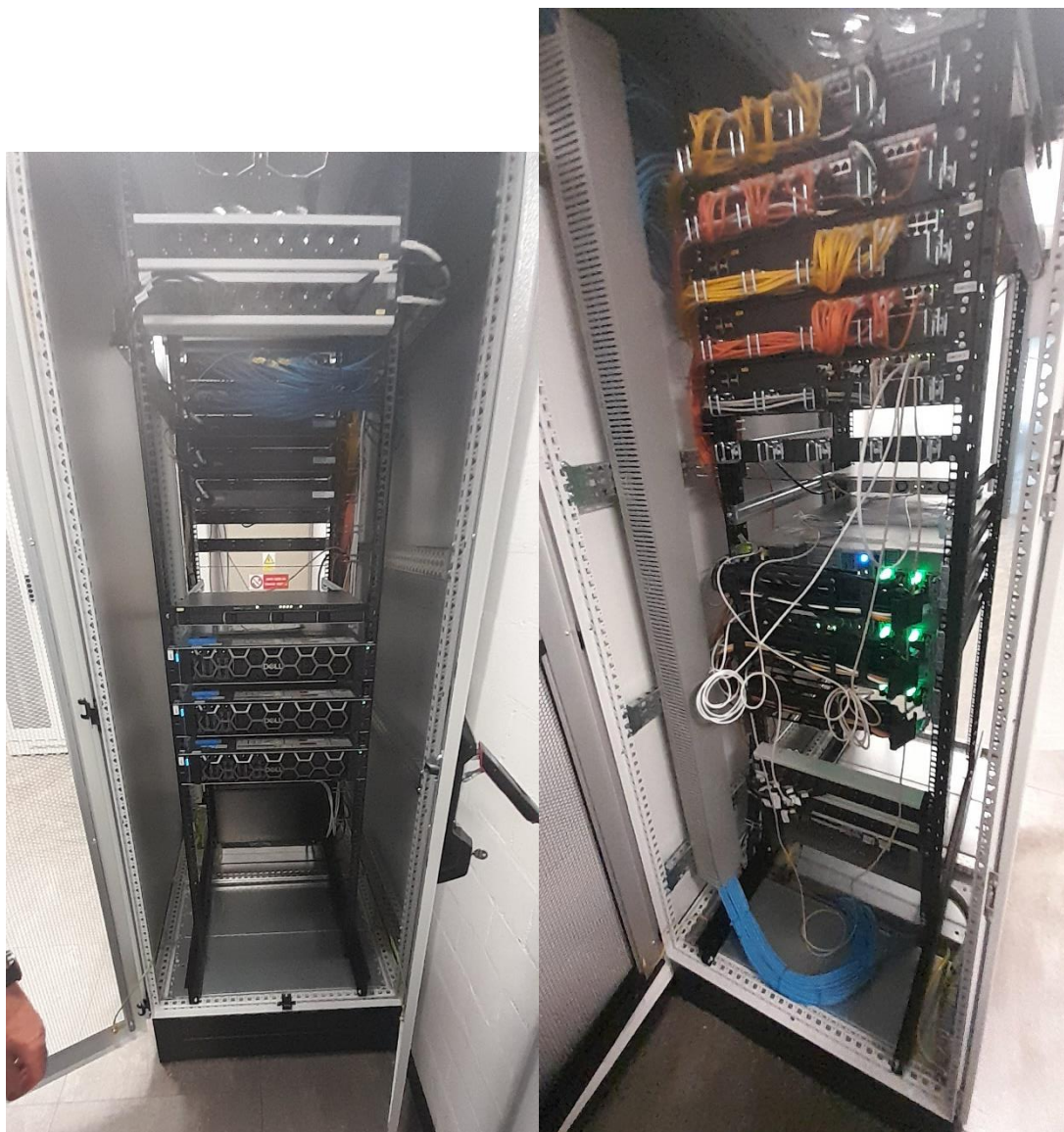
Fig. New cabinets for expanding the 800xA system
