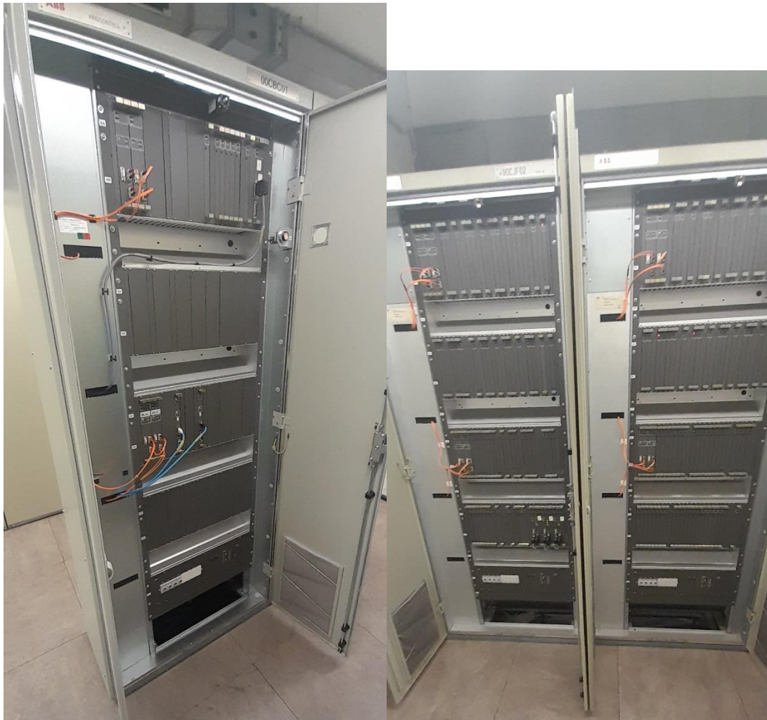
Fig. Cabinets for connecting the retrofit to the Proconotrol P14 system
