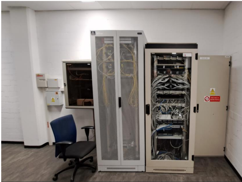
Example of installation of an industrial network in an HV substation (wall-mounted optical switchboard DR2).
