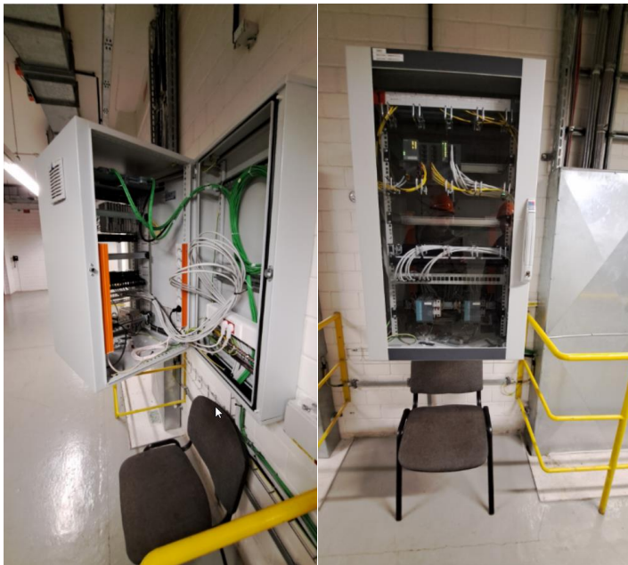
Example of installation of an industrial network in an HV substation (wall-mounted optical switchboard DR2).
